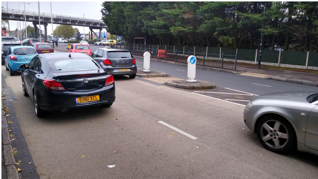
Figure 1 – A118 Main Road, Romford. An uncontrolled pedestrian refuge where pedestrians must find gaps in multiple lanes of moving motor traffic, but which doesn't disrupt those flows.
