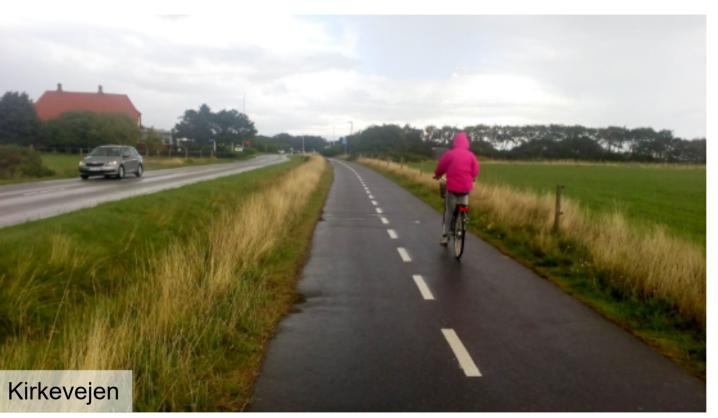
Separation from motor traffic achieved with a verge with a drainage ditch.
