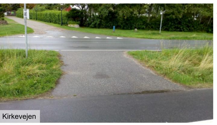
A campsite access with a verge opening to allow access to and from the cycle track.
