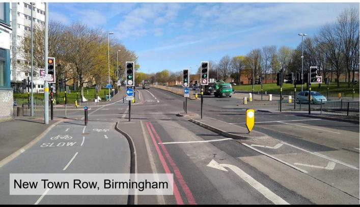
Holding turns to allow a two-way cycle track to run with main road traffic.
