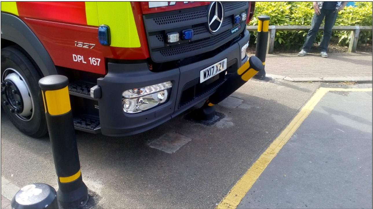
Photograph 5 – collapsible bollard for fire access.
