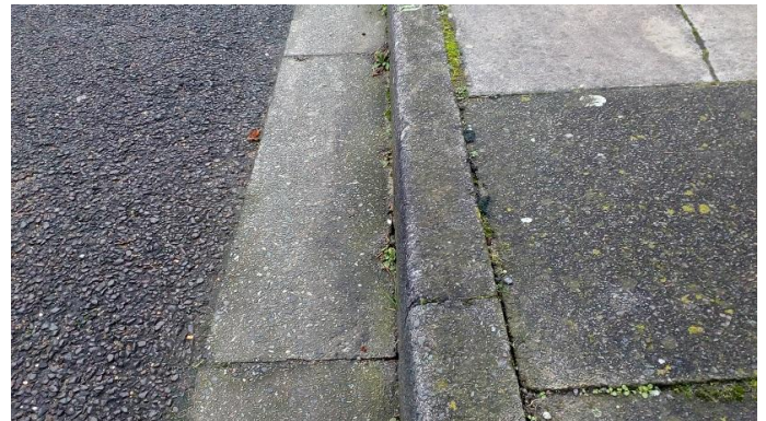
Precast concrete kerb and channel block.
