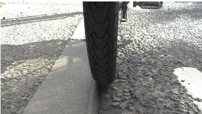
A kerb upstand will “grab” the wheels and throw the rider off their cycle.
