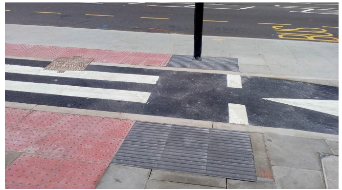
Here, a cycle track is brought up to footway level for a zebra crossing onto a floating bus stop. The area between the red tactile paving and the ramp is flush with the cycle track and so additional “warning” tactile paving (grey) has been added. The layout has become rather fiddly.
