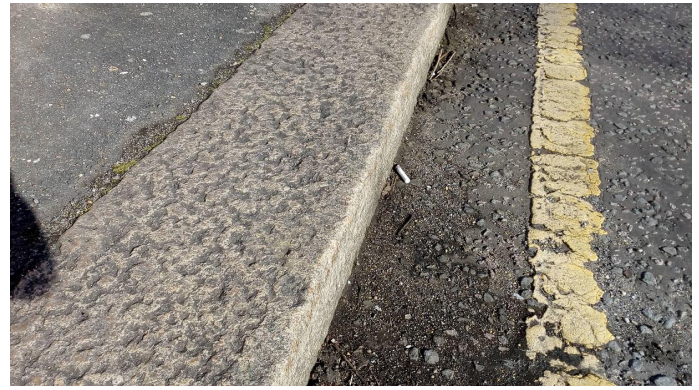
Wide granite kerbs with low upstand (about 50mm) remain in perfect condition while the carriageway surface fails next to it!
