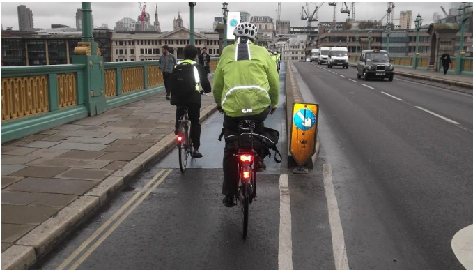
Southwark Bridge, London. The start of a run of containment kerbs protecting the bridge parapet, but providing a cycle track too (containment kerbs behind the keep right sign).
