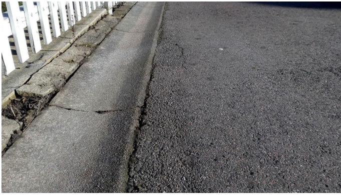
Dished channel at rear of footway to stop water running onto private land behind.
