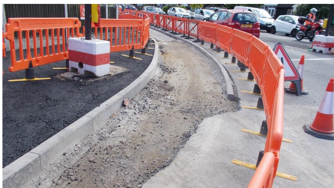
Kerbs being installed, providing the framework for a street retrofit.
