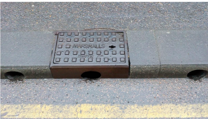
Combined kerb & drainage system access unit.
