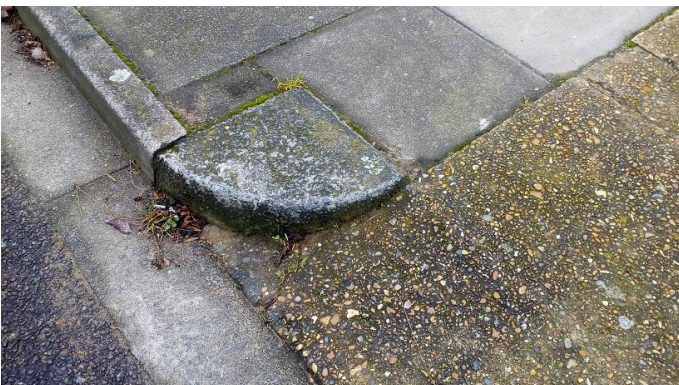
A quadrant being used as a transition between half-battered kerb and a concrete ramped vehicle crossing.
