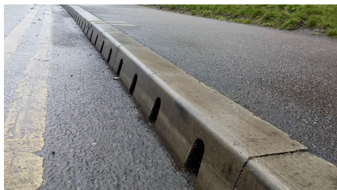
One-piece kerb and drainage system.
