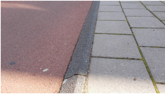
Closer view. Note the textured finish to the surface of the kerb which will help reduce slip risk.
