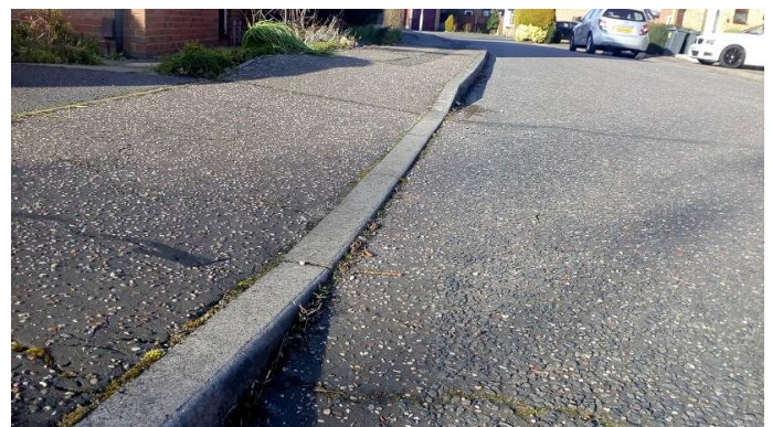
A bull-nosed "dropped" kerb commonly used at driveways and minor accesses. Note the pair of transition kerbs between the dropped and full-height kerbs.
