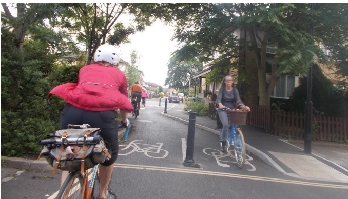
Chaucer Drive, South Bermondsey. Full height half-battered kerbs used on both sides of this link, so there is a risk of pedal strike.
