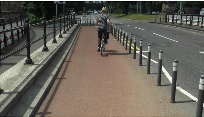
St. Augustine Road, Leicester. Containment kerbs protecting bridge parapets.
