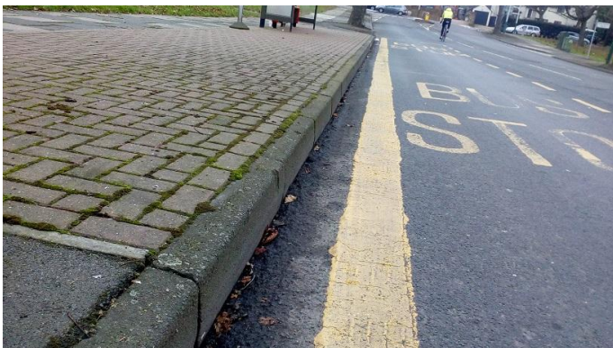
Half-battered kerbs laid with 140mm kerb face at a bus stop, London.
