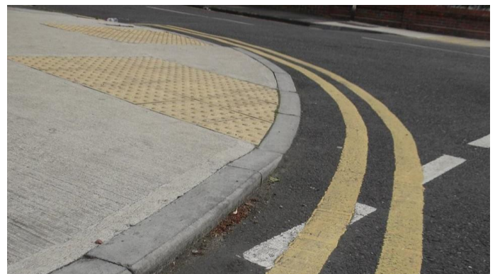
This is part of a raised junction where dropped kerbs are provided at 90° to each other. The kerb face is about 50mm and could be too low for some visually-impaired people to detect.
