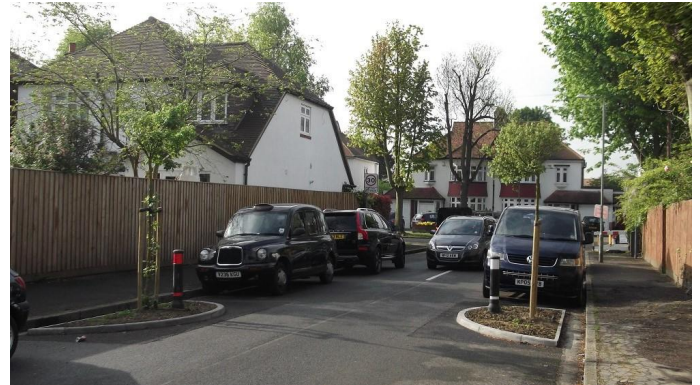
Bridge Avenue, Upminster. Kerbed planting beds within a 20mph Zone.
