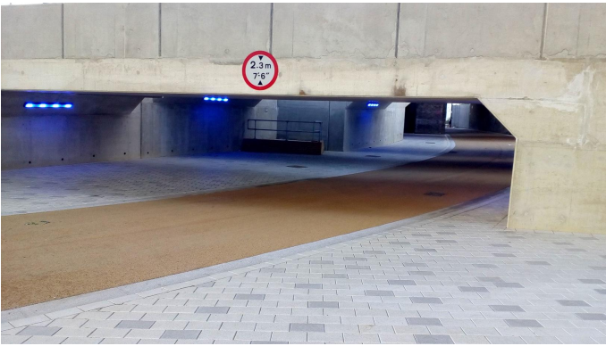
Bolina Road, South Bermondsey, London Footway and cycle track link laid with a level surface which is less helpful to visually-impaired people.
