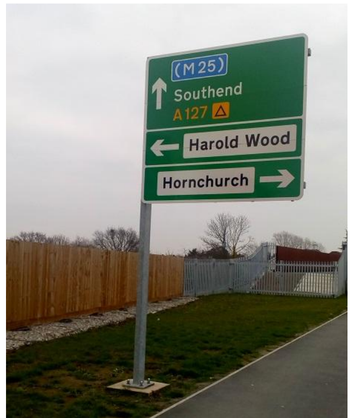
This large trunk road traffic sign has been installed in the verge with a cantilevered frame to avoid a second post placed into the footway.
