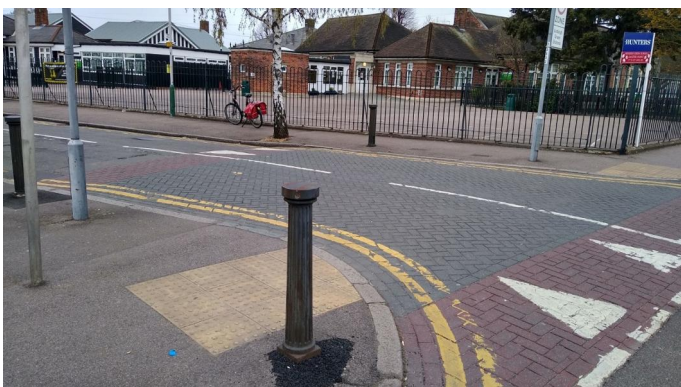
Bollards protecting the crossing points at this side street. The nearest one has been recently reset after being knocked over.
