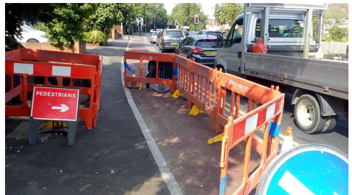
Whilst this worksite has space available to pass, the layout pushes people walking and cycling together.
