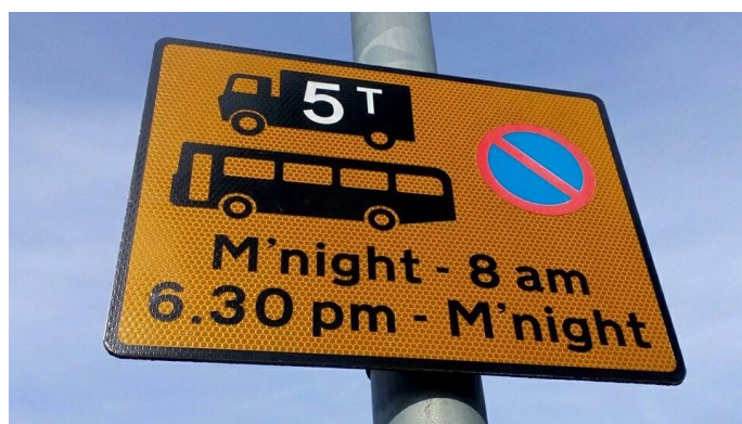
Lorry/ bus overnight parking ban sign attached to a lighting column.
