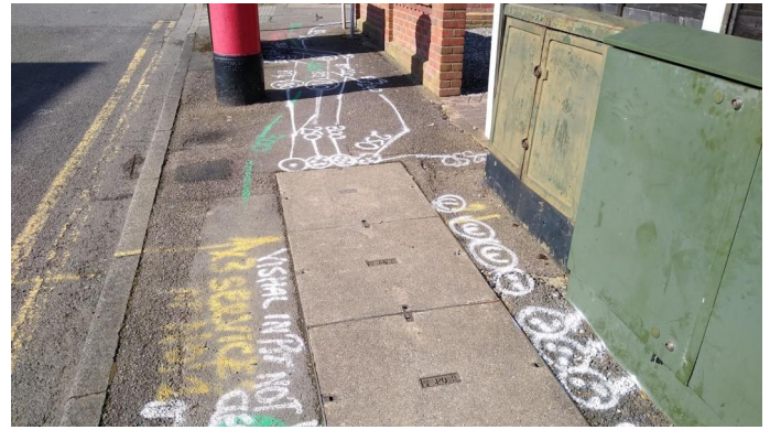
The hidden tangle of buried cables and ducts marked out before repair works.
