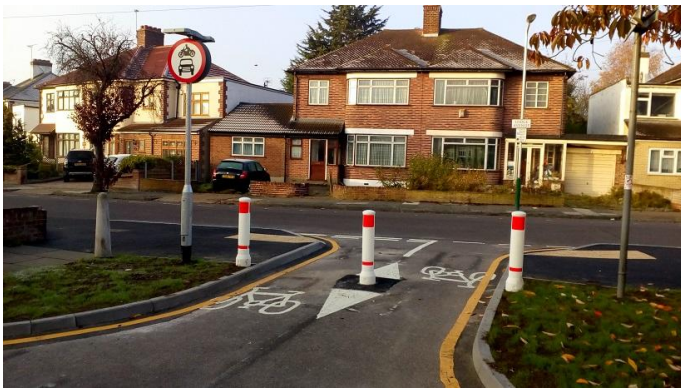
Access control using conspicuous overrunable bollards with 1.5 metre air gap.
