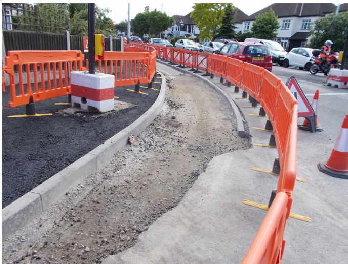
Kerbs being installed, providing the framework for a street retrofit.
