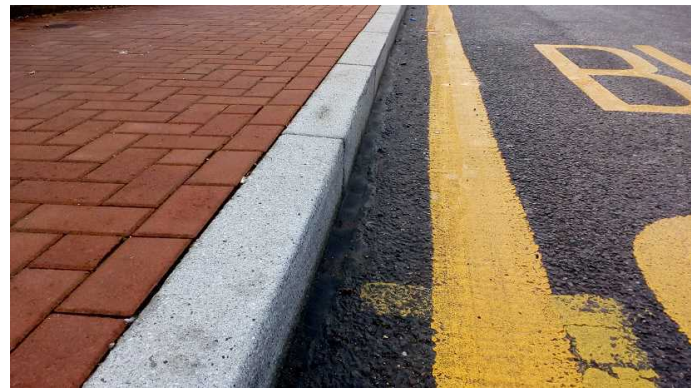
Square kerb used at a bus stop.
