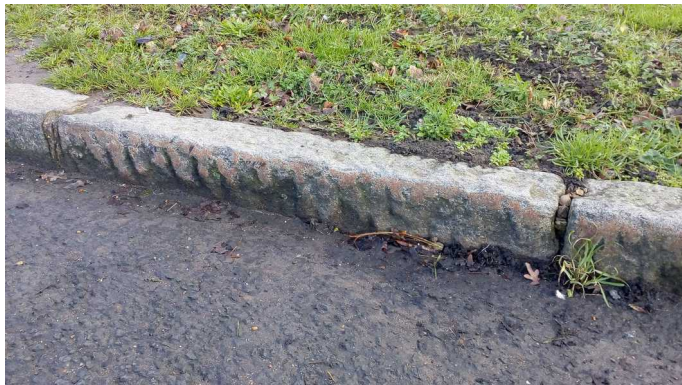
Old granite kerbs.
