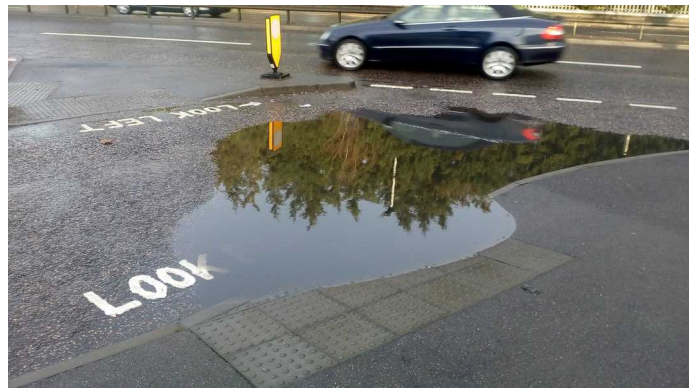
A flooded dropped kerb – not because of a poor dropped kerb installation, but a blocked surface water system.
