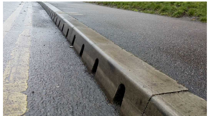
One-piece kerb and drainage system.
