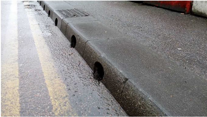
Two-piece, high capacity units.
