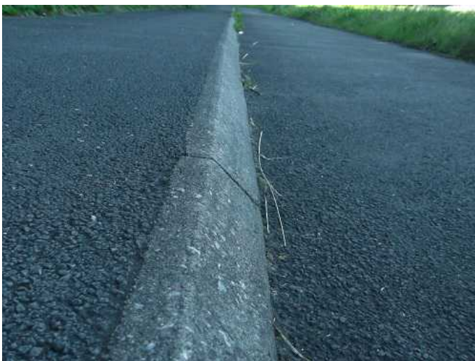
Splay kerb used between a footway and a cycle track on the A48, Port Talbot.
