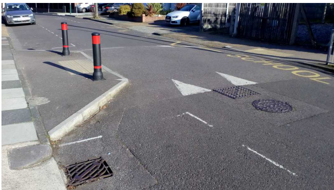
Kerb build-out to create crossing point within a line of parking bays.
