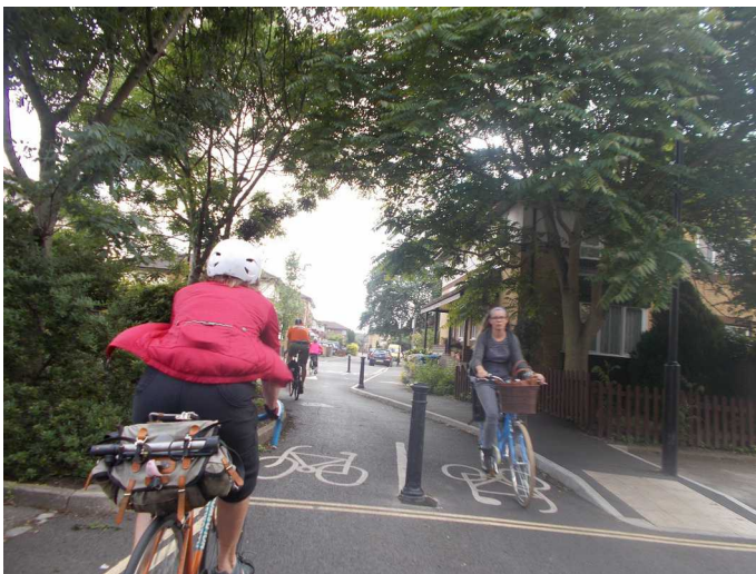
Chaucer Drive, South Bermondsey. Full height half-battered kerbs used on both sides of this link, so there is a risk of pedal strike.
