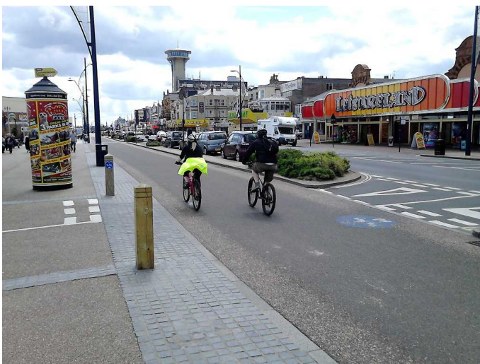
Marine Parade, Great Yarmouth, A low, square, granite kerb is used on both sides of this carriageway-level cycle track, so there is some risk of catching wheels. A wide “island” area provides space for other uses.
