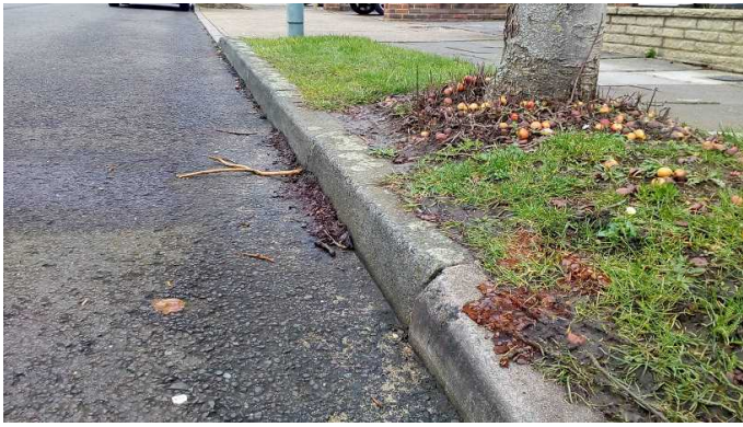
A half-battered kerb with most common dimensions to be found on the street.
