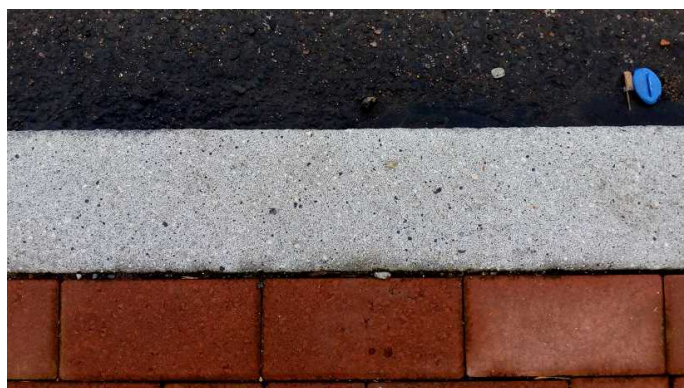
Conservation type kerb with dark granite flecks.
