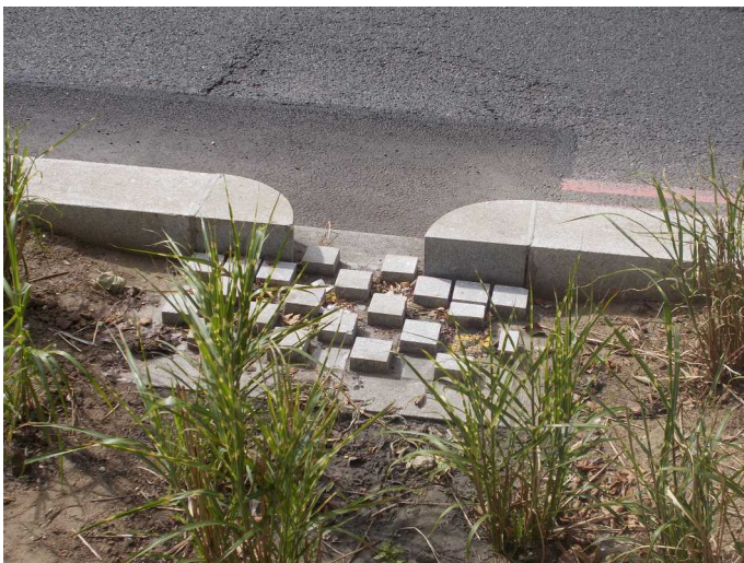
A simple inlet from the carriageway into a planted storage/ infiltration area. A gap in the kerb run is finished with quadrant kerbs and a flush kerb between. The granite cubes slow the speed of the water as it enters the feature.
