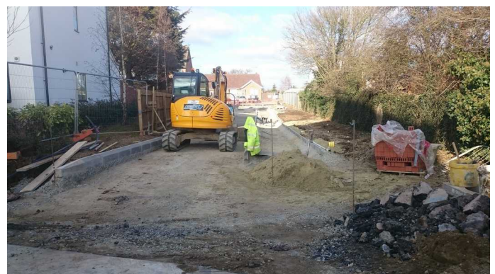
New kerb lines being installed. Note that they are laid on a concrete bed which is in turn supported by a structural layer which extends beyond the kerb line to provide proper support.
