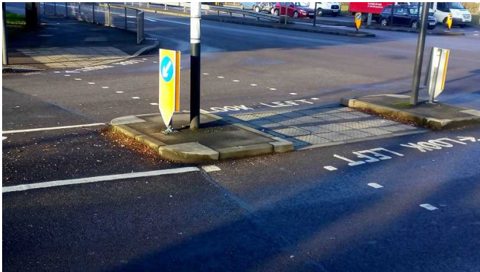
Quadrant kerbs being used on traffic approaches to pedestrian refuge and corner kerbs being used on pedestrian area.
