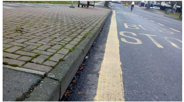
Half-battered kerbs laid with 140mm kerb face at a bus stop, London.
