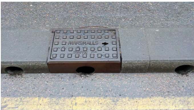
Combined kerb & drainage system access unit.
